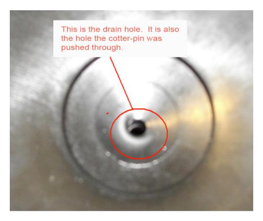
Use anything you have available to clear out the hole. Example: Screw Driver, Stick, Q-tip etc.... Once the drain is cleared, re-insert the screen and cotter pin.
